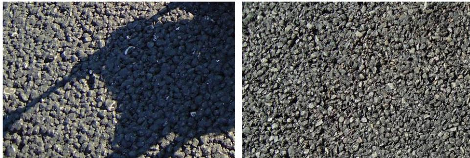
Figure 5 Surfacing with slag (left) and natural aggregate (right)
